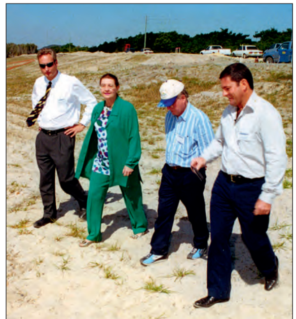
Scott Hutchinson; Cr Lynne Beck, Mayor Tweed Shire Council; Dr Jim Gallagher, Chairman Northern Development Task Force; and Don O'Rourke, Consolidated Properties, celebrate the commencement of construction of Casuarina Beach on September 11, 2000. Photo: Andrew Carille
